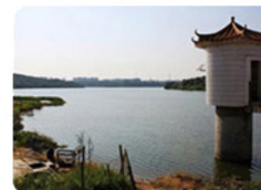
Reservoir and level
