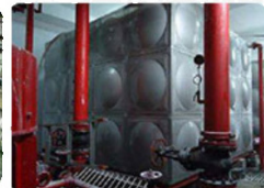
Fire and tank water level
