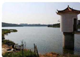
Reservoir and level
